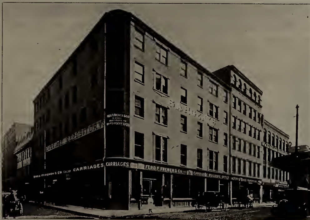
FACTORY AND WAREROOMS OF FERD. F. FRENCH & CO., Ltd., Carriage Builders,
